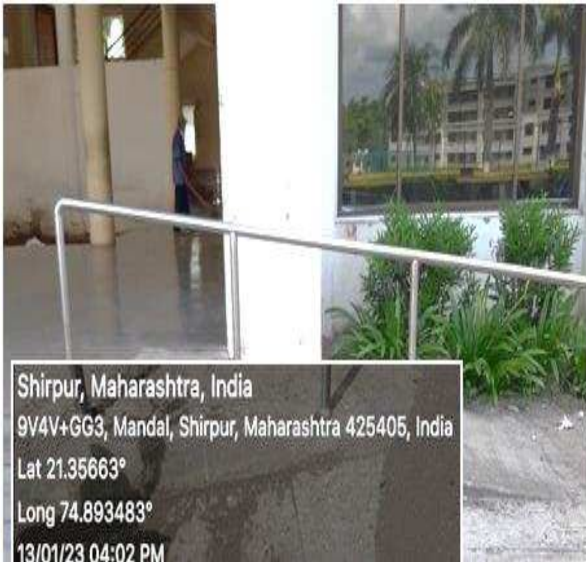
Ramp for easy access to Classrooms
